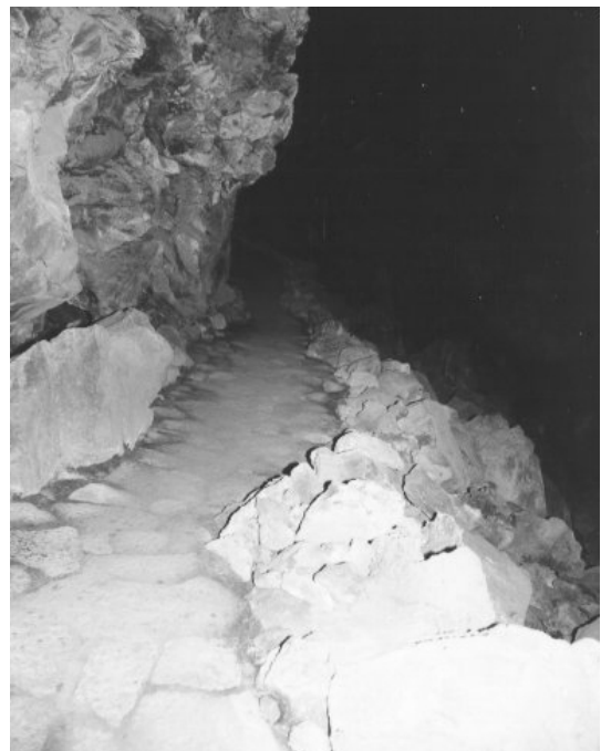
Figure 14. Dry and wet mortar was packed into spaces between slabs. The dry mortar was then wetted to cement the basalt slabs in place. (Photo by Kelly Fuhrmann)
