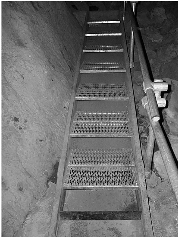
Figure 3. New stairs in Skull Cave made of galvanized steel with \frac{1}{2} -inch mesh. Also notice the steel tray under the structure and catchment trough at the base of the stairs (photo by Kelly Fuhrmann).
