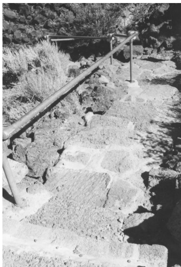
Figure 16. Photograph taken in August of 2000 from the same location as Figure 15. All loose debris was removed, new basalt lava slabs added, and the trailhead renovated. (Photo by Kelly Fuhrmann)
