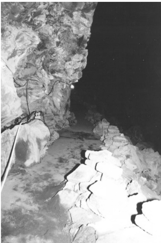
Figure 12. A basalt sand base was added over the original trail tread material. (Photo by Kelly Fuhrmann)
